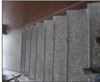
Photo of the inside of the main production hall anti slippery bands.JPG
