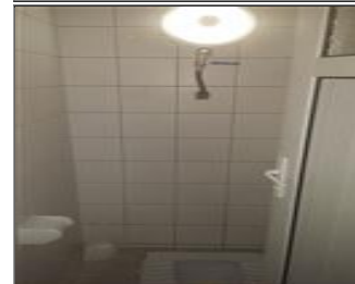
Photo of the sanitary facilities Toilet (3).jpg
